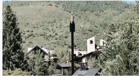
Custom-designed slimline poles accommodate small cell nodes.
