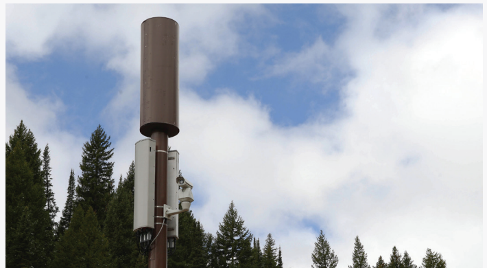
Small cell nodes installed on a slimline pole.
