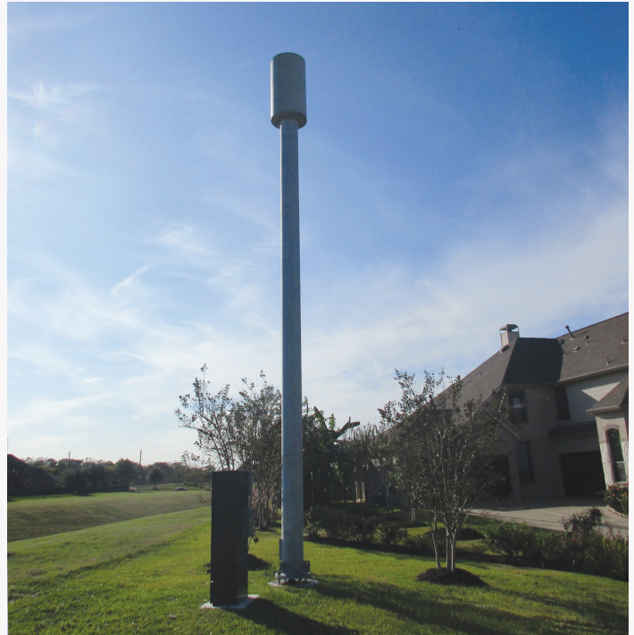
Small cell node installed on a slimline pole.
